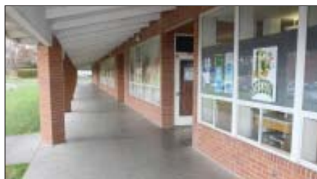
All outdoor breezeways will be replaced with interior hallways. This allows for more classroom space, improves efficiencies and eliminates exterior doors for safety.
